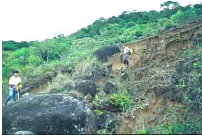
Figure 4. Erosion, Bom Abrigo Island. Photo: Marcelo R. Duarte.
