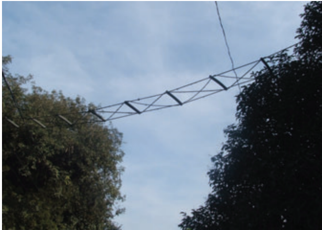
Figure 2. Rope overpass constructed with four 12 mm ropes interlaced and rubber hose to form ladder steps in Lami district, Porto Alegre municipality, southern Brazil. Photo: João Cláudio Godoy Fagundes.
